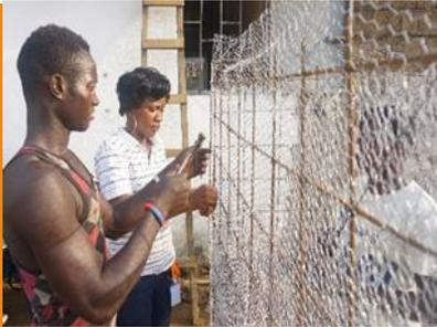
*Fabricating the metal cage, that is, the structural support for the tank. Metal cages can be fabricated off-site for mass production and cost-saving purposes.*
