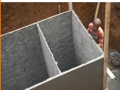
*Ferrocement septic tank under construction in Yopougon, a suburb of Abidjan (Cote d'Ivoire).*
